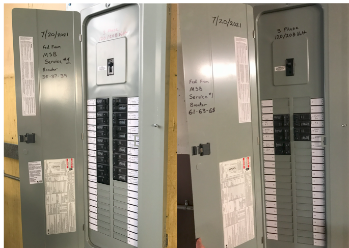
Figure 19 Branch Panels W and M fed from MSP in existing Shop Building
