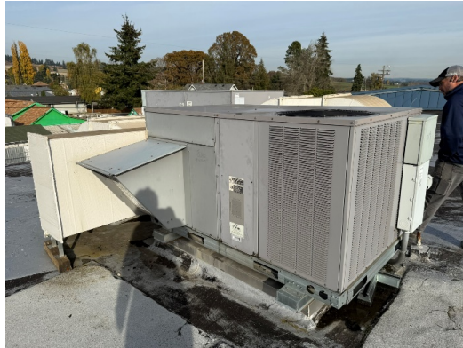
Figure 2 There are four rooftop air handling units that past expected useful life.
