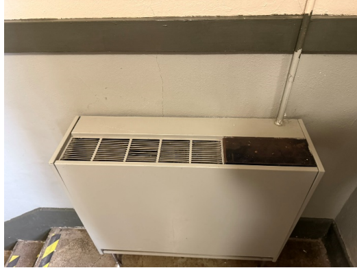
Figure 7 The unit ventilators serving the admin building are not functional and past end of useful life.
