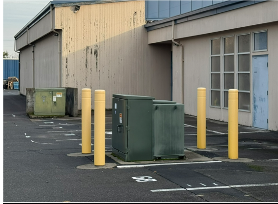
Figure 11 Pad-mounted Transformers
