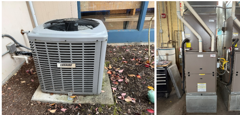
Figure 3 The classrooms are served by residential style furnaces and outdoor condensing units.
