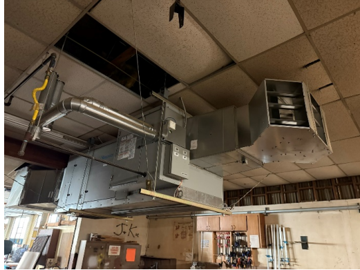
Figure 4 Gas-fired HVUs serve the CTE classroom spaces. These units appear to be in good condition overall and upgrades may not be necessary.
