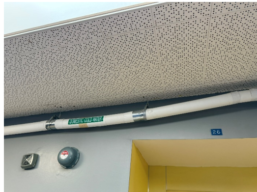
Figure 1 To upgrade the chemistry classroom, cold water piping has been run along the ceiling in the hallways. It is at risk of failure and could cause large flooding issues in the hall.
