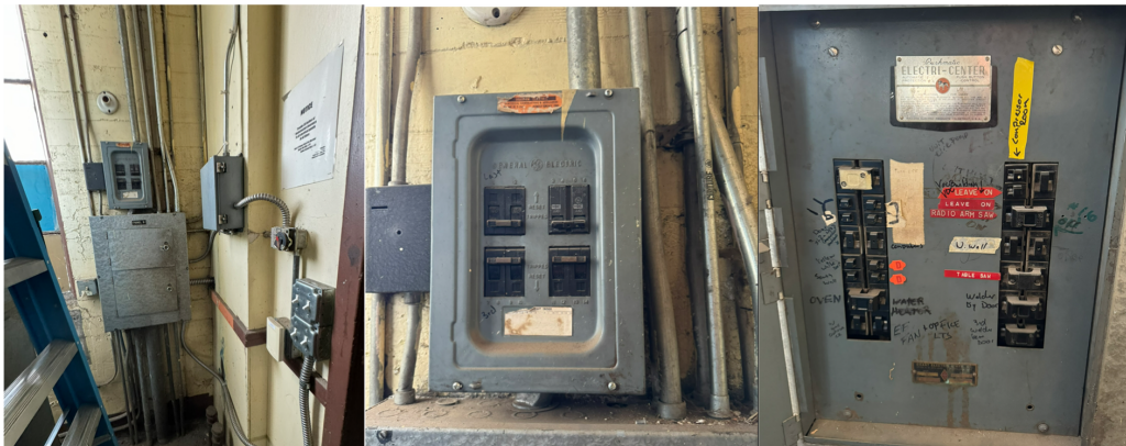
Figure 20 Load centers in existing Shop Building
