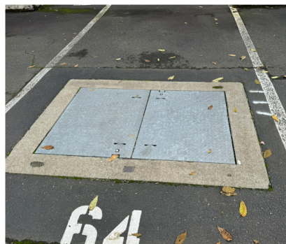
Figure 10 Underground Vault
