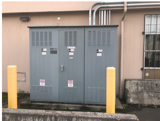
Figure 12 Existing Electrical Service #1 (MSP)
